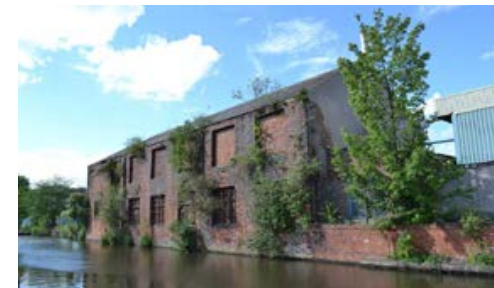
4. View of canal side warehouse
