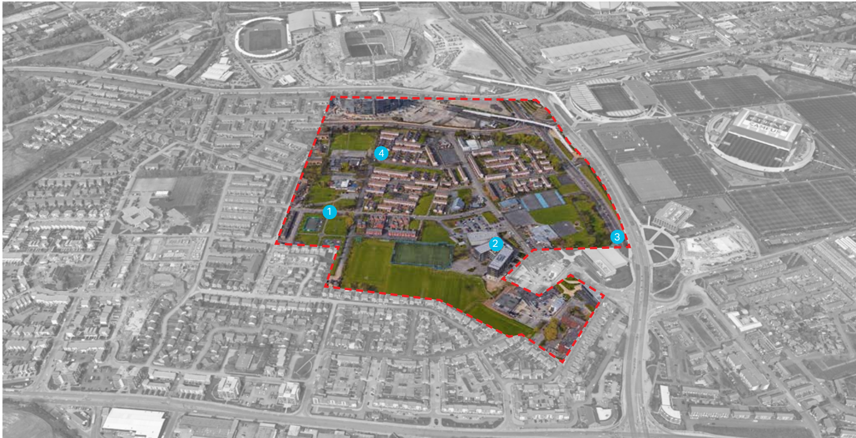
Figure 7.11 Aerial view of the regeneration area from south
