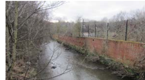
3. View of River Medlock looking South
